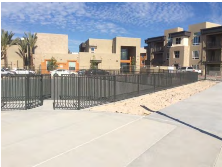
1. Stylus Park Under construction – Dog Park
