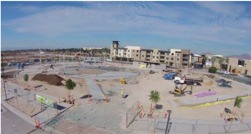
1. Stylus Park under construction – air view
