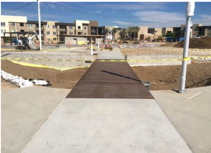
1. Stylus Park under construction – Bridge to splash plaza and restroom.
