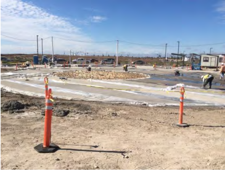
1. Stylus Park under construction – splash pad pipework
