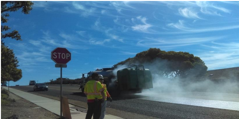
Major Street Projects - $9.1M
