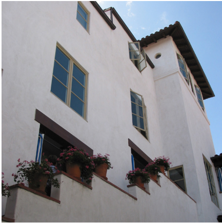
Terraced walls with red brick cap and simple door header provide Spanish detail to a simple building form and basic-trimmed windows.
