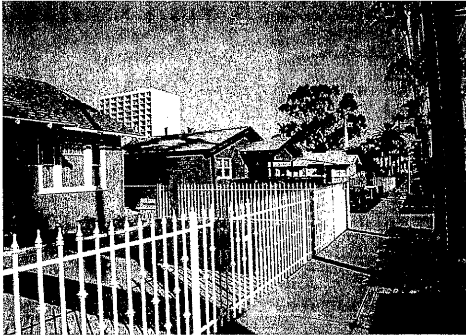
Figure 8. Streetscape view of block of modest Craftsman style single family residences, west side of 300 block of Del Mar Avenue.
