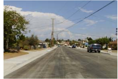
Oxford Street Improvements
