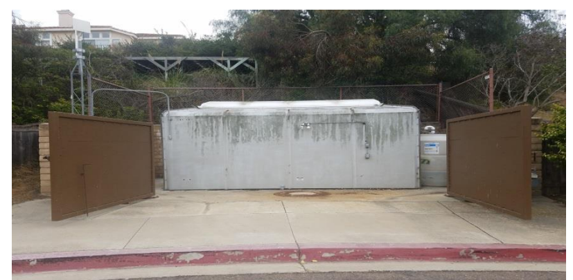
Parkside Drive Lift Station - $1M
