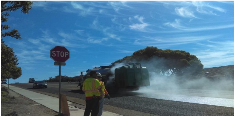
Major & Minor Pavement Rehab - $7.4M
