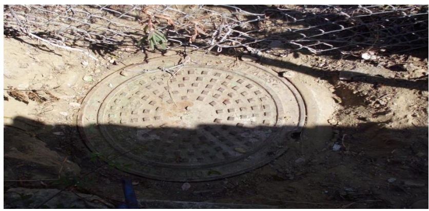
Manhole Rehab & Inspection - $500k
