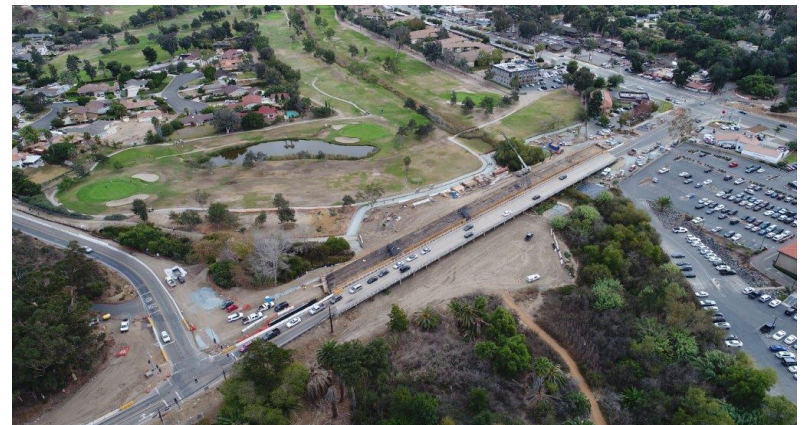
Willow Street Bridge - $1.6 million
