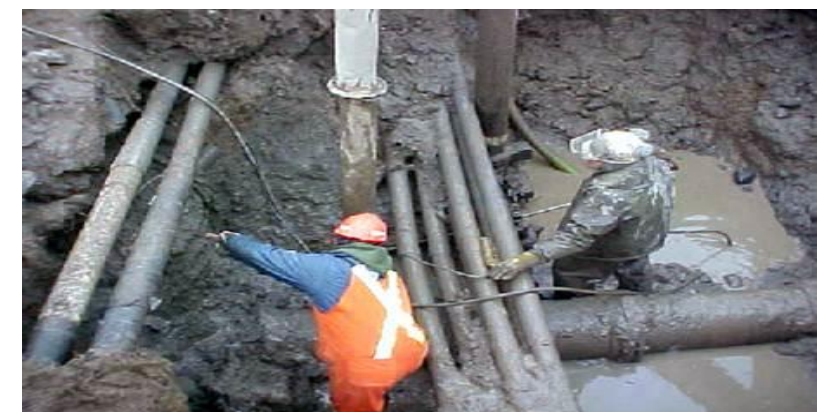
Sewer Pipe Rehab - $300k
