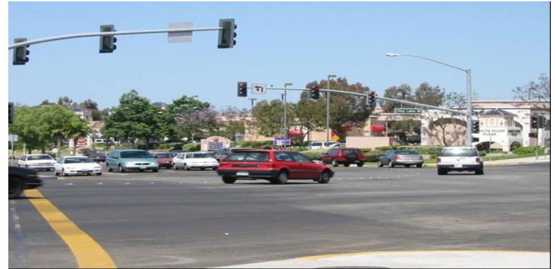
Traffic Signal Projects - $2.7M
