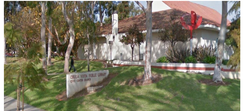
Civic Center & South Libraries Repairs - $1.5m
