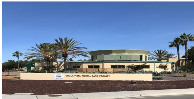
Other Public Building Repairs - $3.1 million
