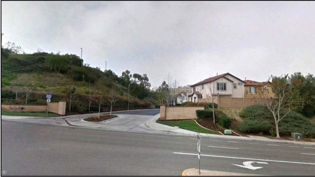
View of Existing East Tower from Intersection of Paseo Ladera and Mandeville Drive Facing West
