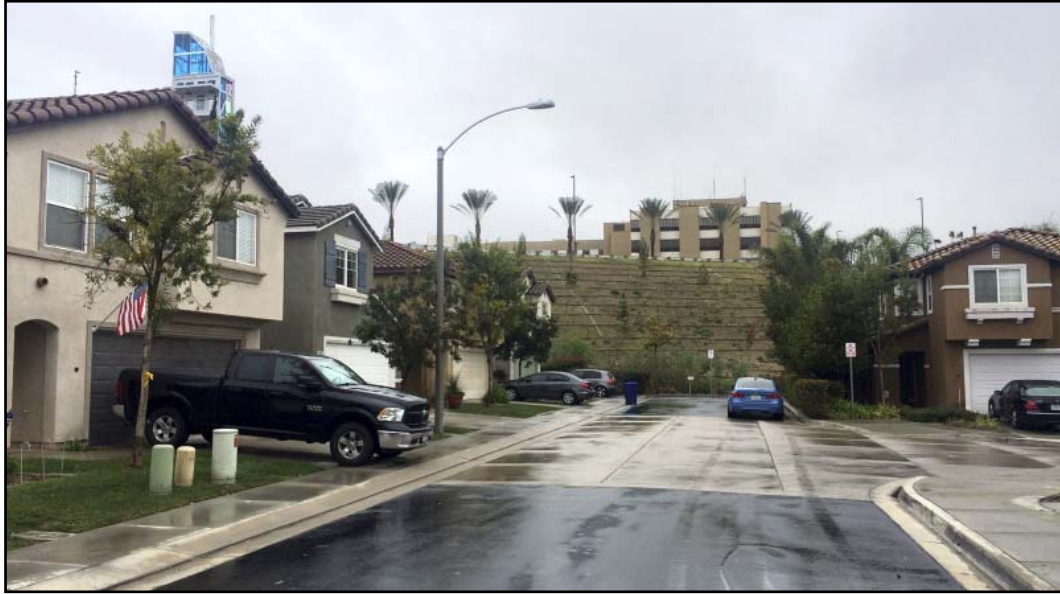
View of Existing East Tower from Caminito Cumbres Facing West
