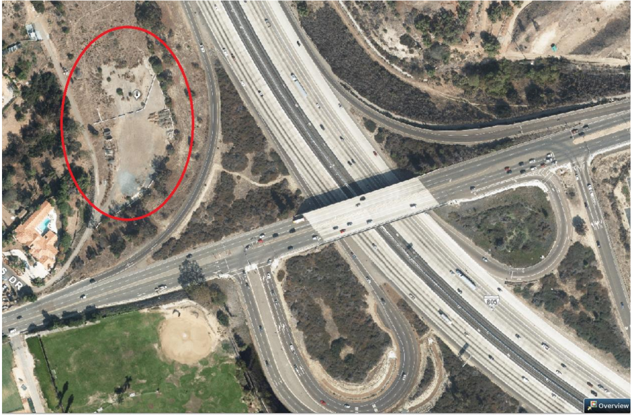
CalTrans Sale- 805 Express Lane Project. NW corner of Hst and I-805
