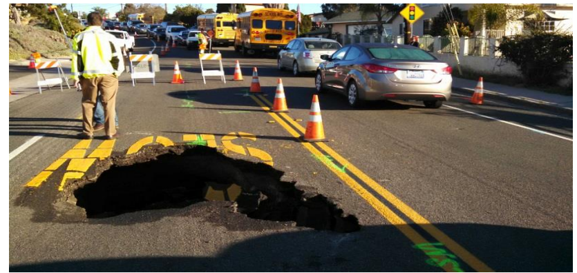
Storm Drain Rehab
