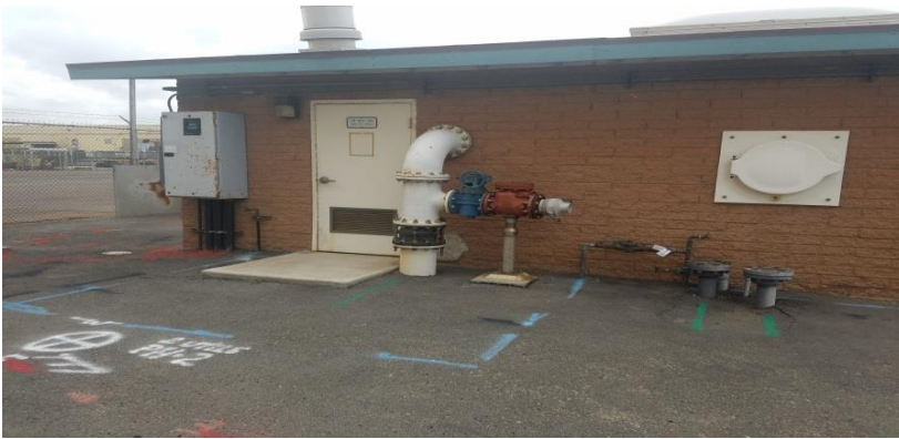
G Street Pump Station Upgrade
