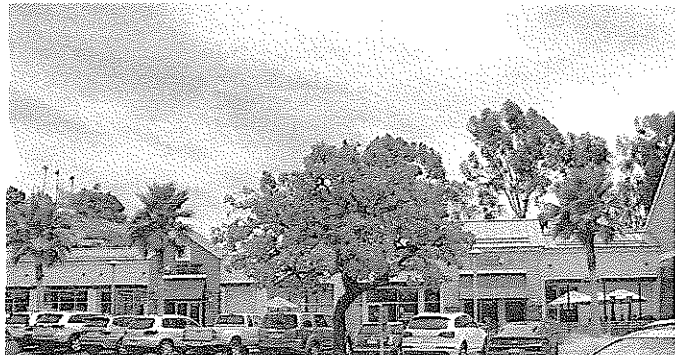
EXISTING SHOPS 1A NORTH ELEVATION
