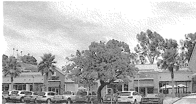
EXISTING SHOPS 1A NORTH ELEVATION
