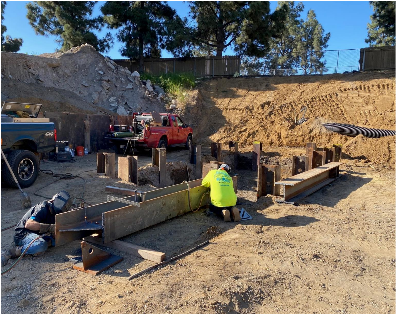
Figure 2 - Reconstructed Slope and Welders Beginning the Shoring Construction
