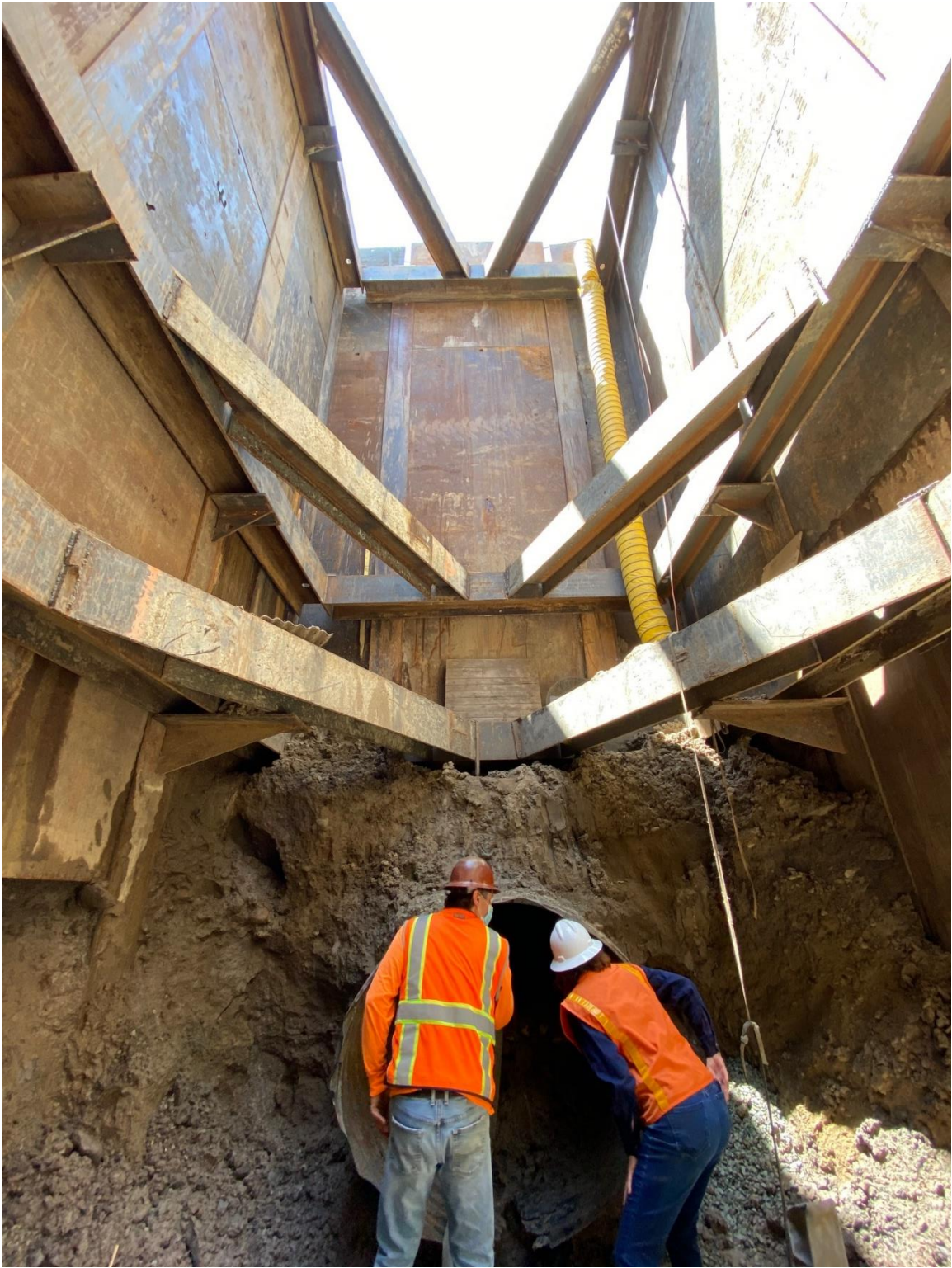
Figure 4 - Examination of the pipe
