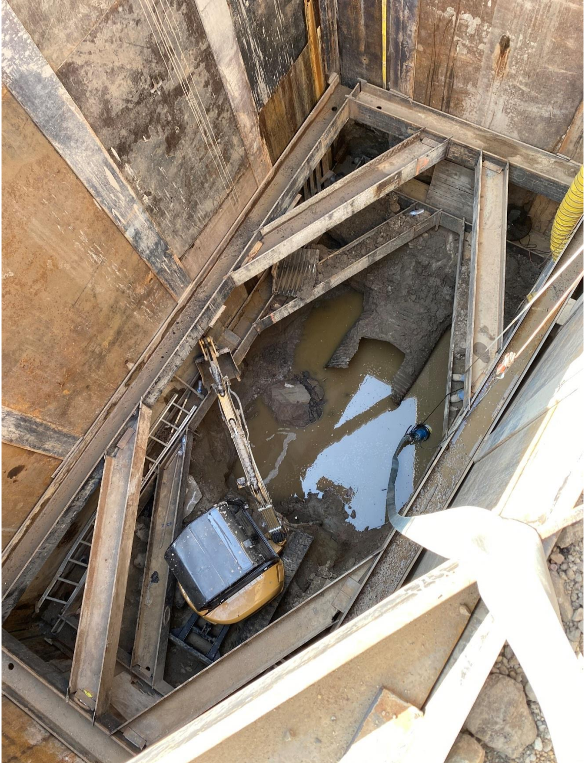
Figure 3 - View into Excavation Pit Showing Shoring and Existing CMP
