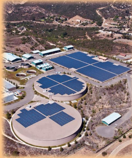
Twin Oaks Valley Water Treatment Plant $179 million
