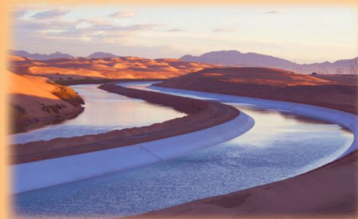
All-American & Coachella Canal Lining Projects $447 million ($190 million from Water Authority)
