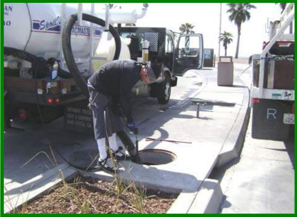
Access Pre-Treatment Chamber by Removing Manhole or Grate Cover
