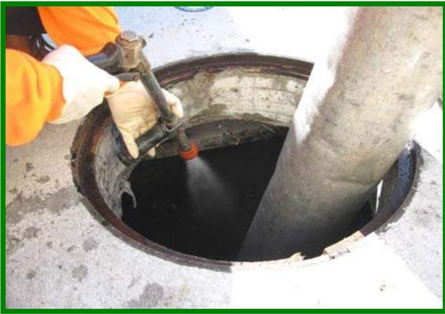
Vacuum out the Sediment Chamber
