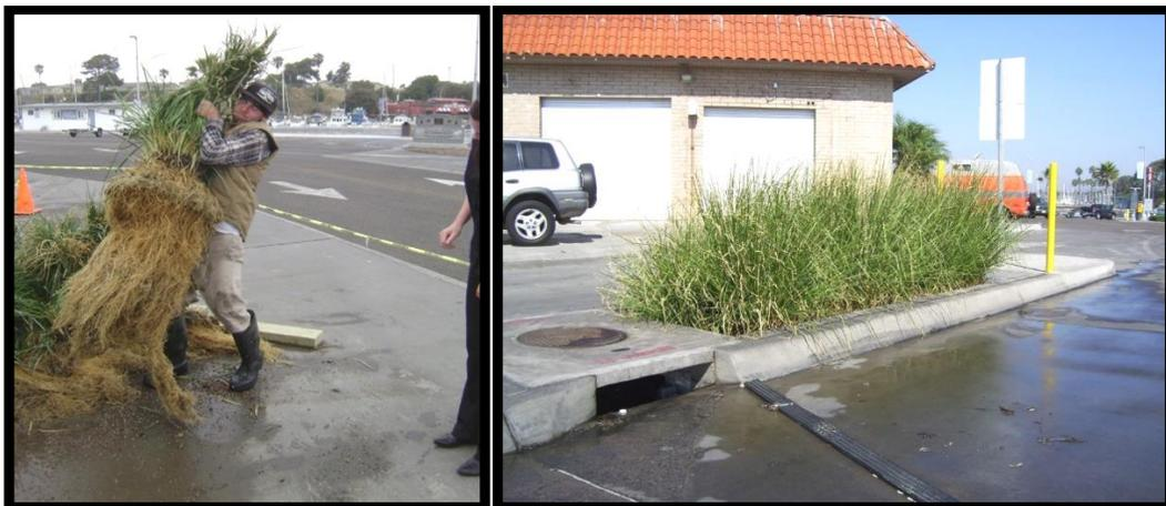
6. Biofiltration BMPs must be designed to prevent erosion, scour, and channeling within the BMP.
