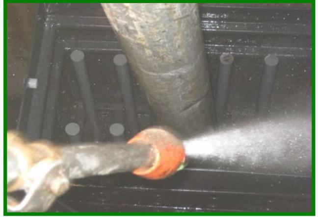
Spray Down and Clean Cartridge Filter Housing
