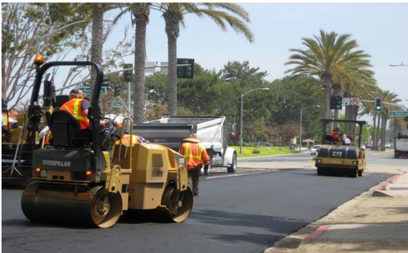
Pavement Rehabilitation - $6 million
