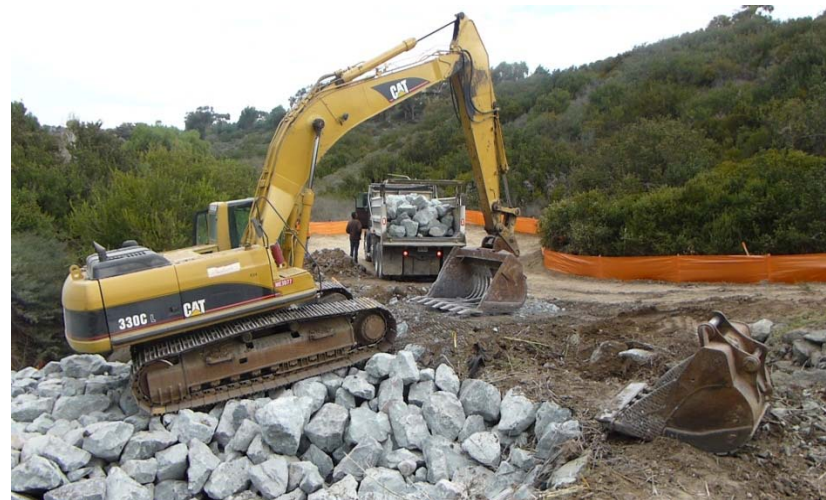
Storm Drain Repairs - $1.6 million
