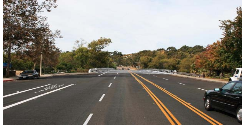
Willow Street Bridge - $7 million
