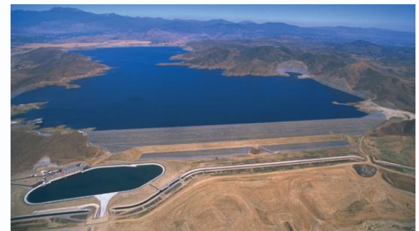
Metropolitan Water District Diamond Valley Lake
