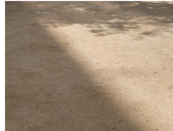
STABILIZED DECOMPOSED GRANITE AT GATHERING AREAS
