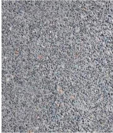
EXPOSED AGGREGATE CONCRETE AT BBQ AREAS
