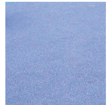
POURED IN PLACE RUBBER SURFACING AT FITNESS AREA
