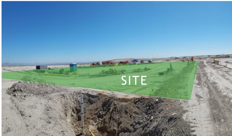
VIEW INTO SITE FROM NORTHEAST CORNER ALONG STRATA ST.
