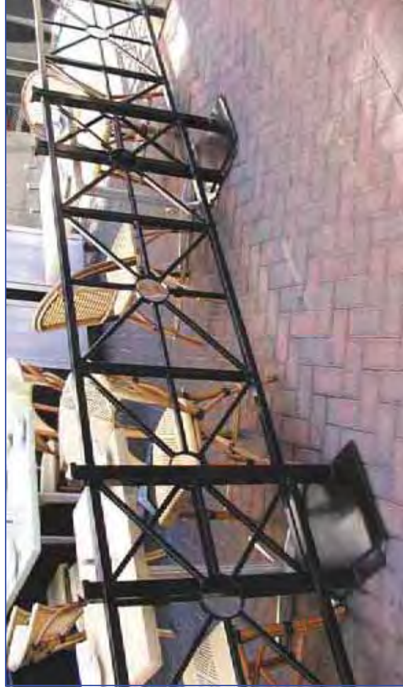
Figure 5: A great example of the outdoor sectional fencing that is linked together with a great design and has a low profile stanchions.
