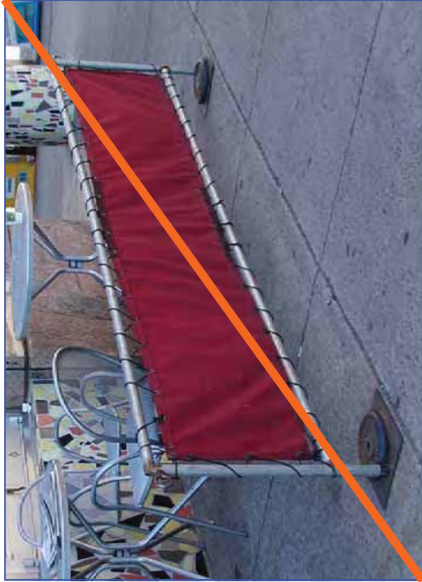
Figure 6: Fencing with fabric inserts are not permitted to be used as part of the barrier.
