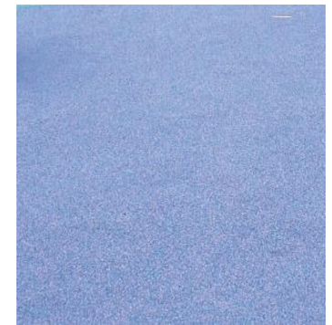
POURED IN PLACE RUBBER SURFACING AT FITNESS AREA
