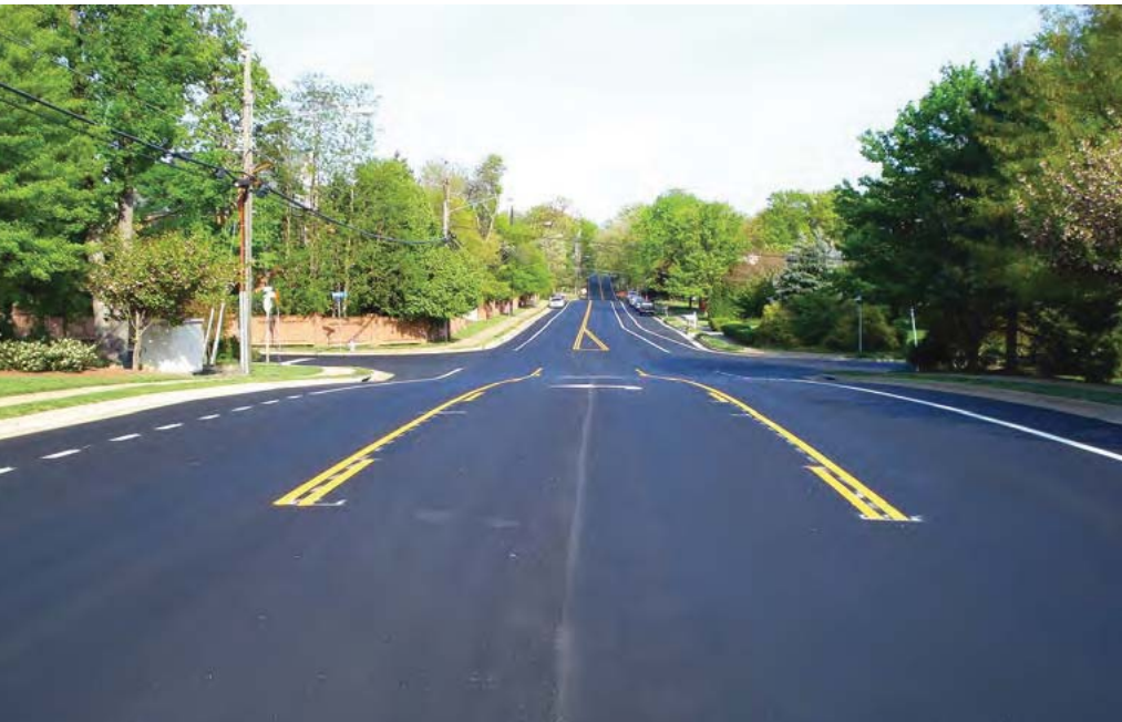
Figure 23. Transition from 3-lane to 2-lane Cross Section, Oak Street, Merrifield, VA Photo Credit: Virginia DOT
