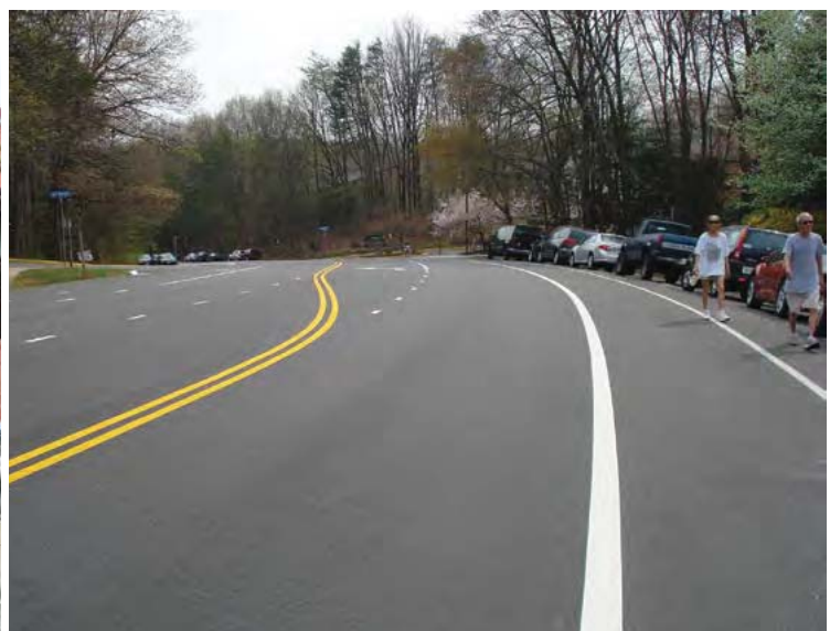
Figure 15. Pedestrians Buffered from Traffic in Reston, VA Photo Credit: Richard Retting
