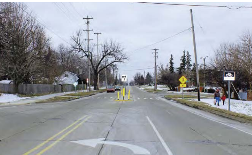
Figure 8. Mid-block Pedestrian Refuge Island Photo Credit: Jennifer Atkinson
