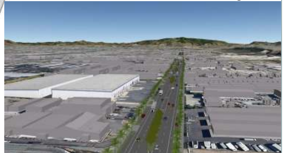
From Industrial Blvd. looking East
