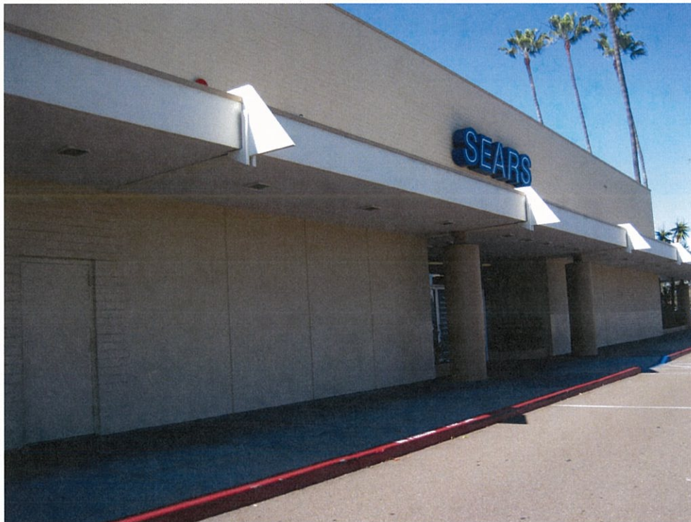
Figure 2-13: East façade showing the enclosed display windows.
