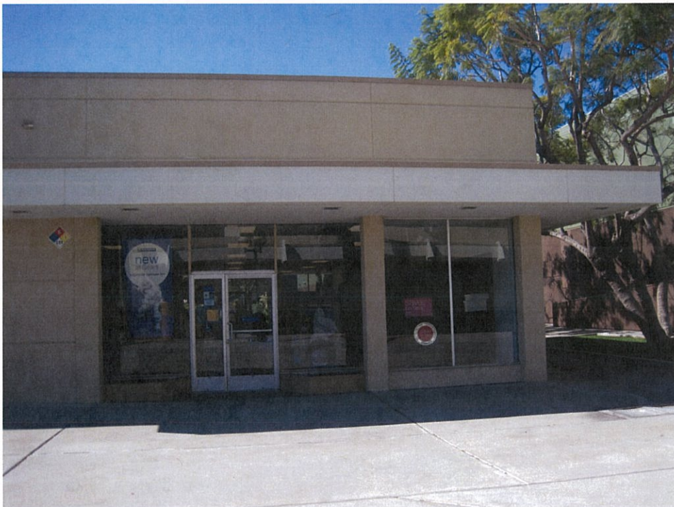
Figure 2-15: Looking west at the Sears Auto Center service entry.
