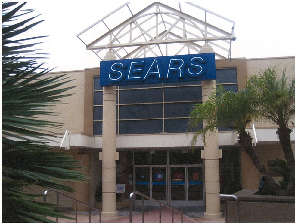
Figure 2-8: Renovated southwest entry showing notched canopy at entry and 1980s open-framed gabled entry structure.
