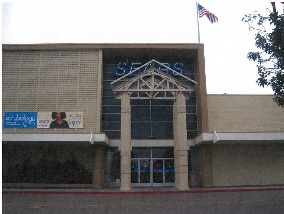
Figure 2-3: View of renovated entry at the north façade with contemporary signage and original large charcoal gray Mirawal panels. The entry canopy has been notched at the storefront entry for the 1980s open-frame gabled canopies.
