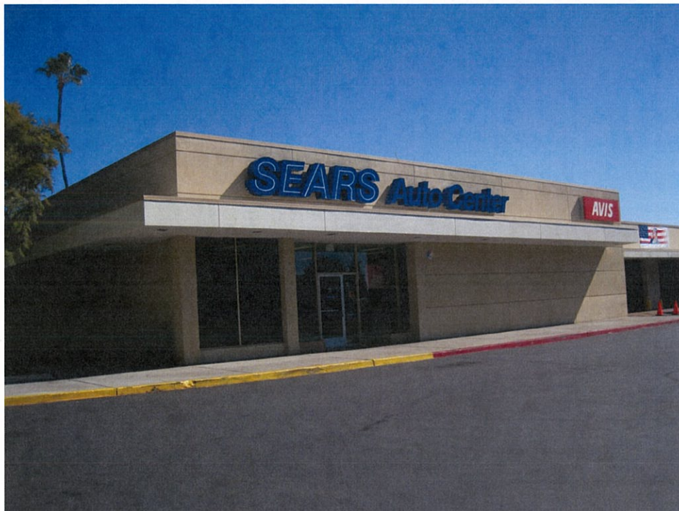
Figure 2-17: Looking southeast at the Sears Auto Center building. The north façade's original storefront windows and original brick wall to the right of the west storefront are no longer extant. All original signage have been replaced with contemporary ones.
