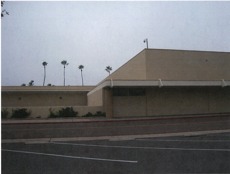
Figure 2-12: Southeast corner showing enclosed walkway.
