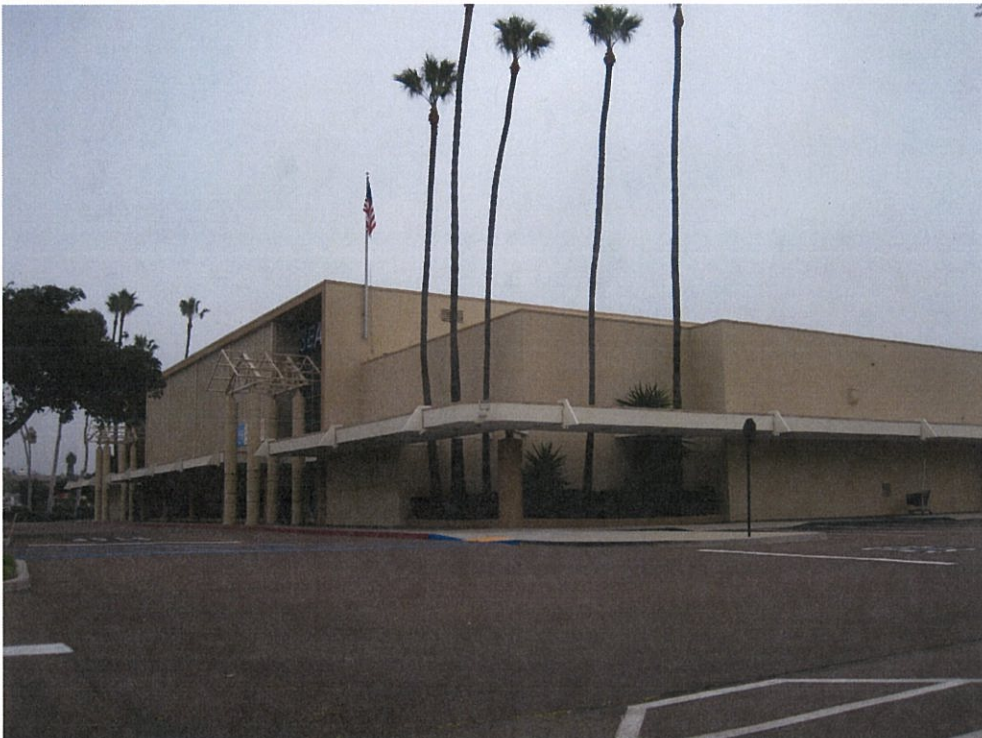
Figure 2-5: Looking southeast at the Chula Vista Sears building.
