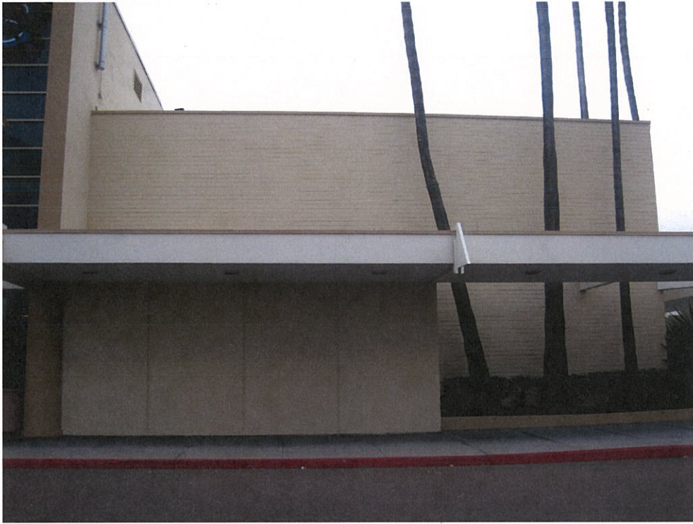
Figure 2-4: Detail of original storefront display windows (now enclosed) and planters at the northwest corner.
