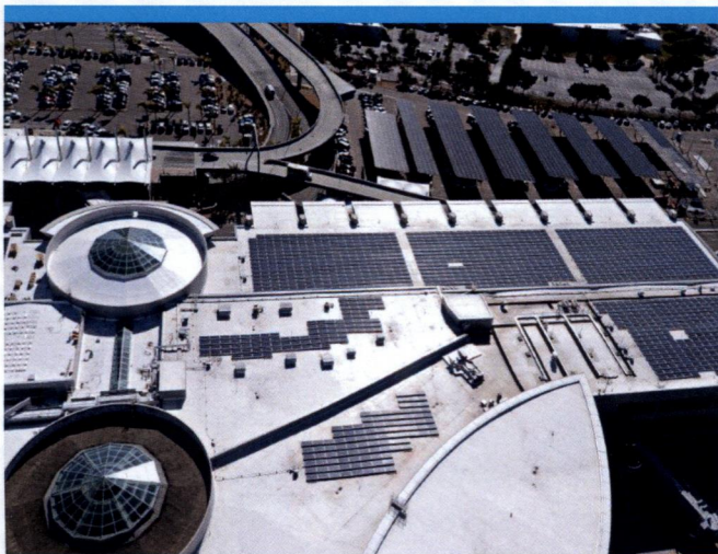
Solar panels on terminal roofs and carports in parking lots generate electric power for the airport.
