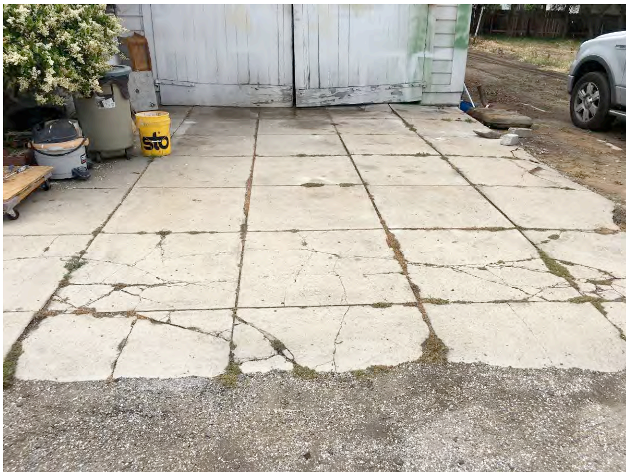
Photo 20: Concrete drive in front of the west wing garage.
