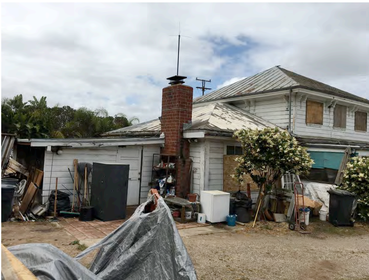
Photo 2: View southwest of the east wing with shed roof addition and brick chimney.
