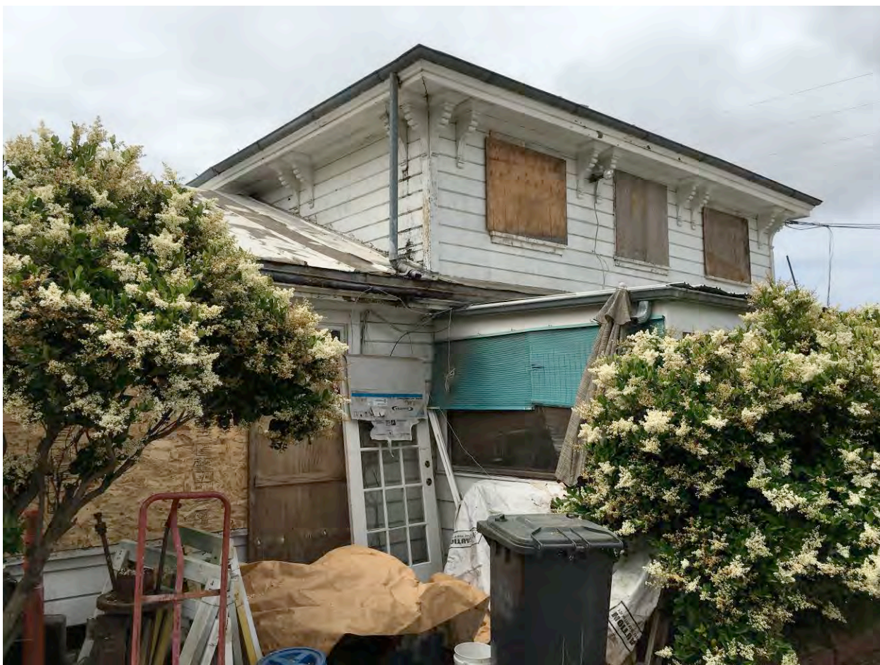
Photo 23: View southwest of the north elevation where the central block and the west wing connect with the framed porch appended to the facade.
