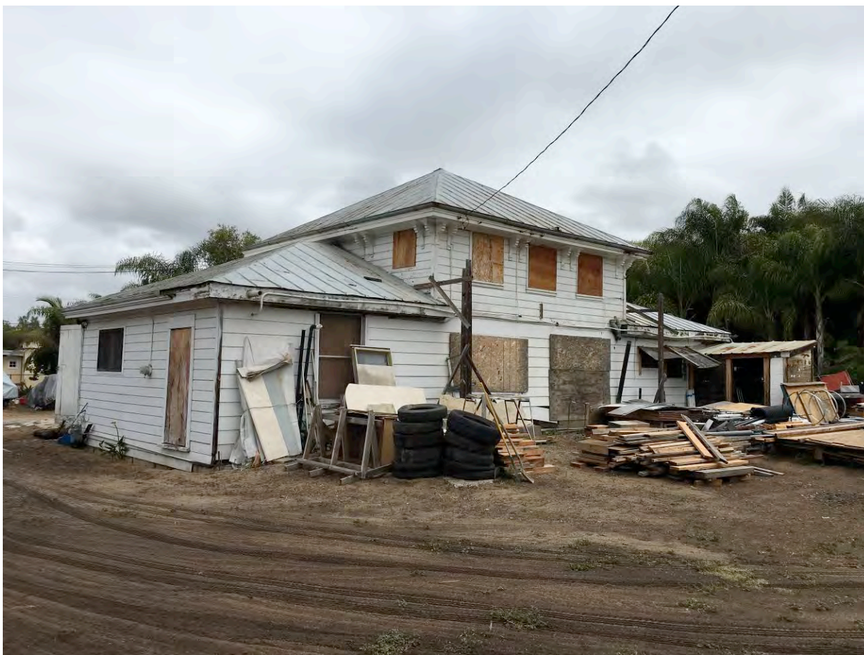
Photo 12: View northeast of the south elevation (at right) and the rear façade of the west wing (at right).
