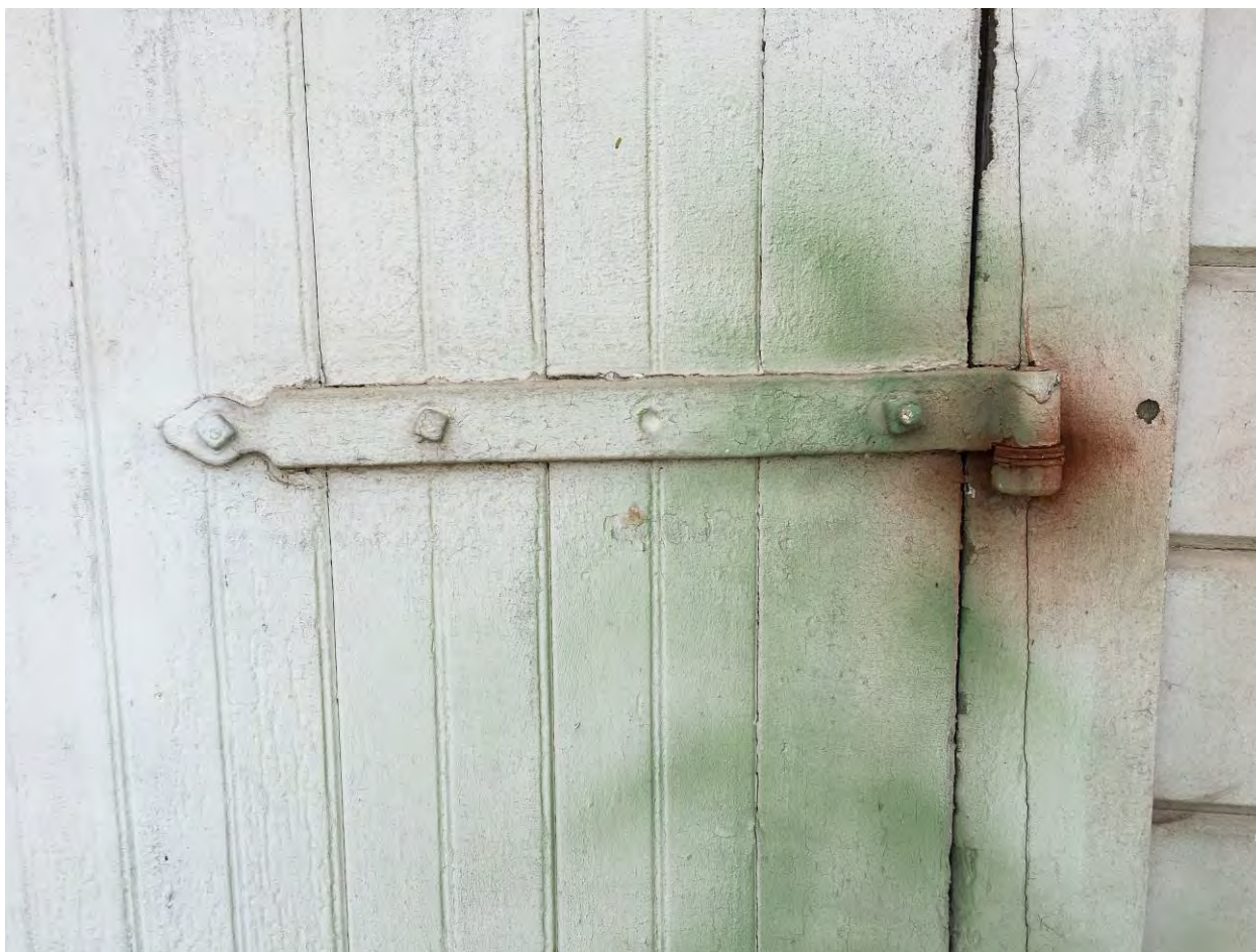
Photo 19: Detail of a typical hinge at the garage door.
