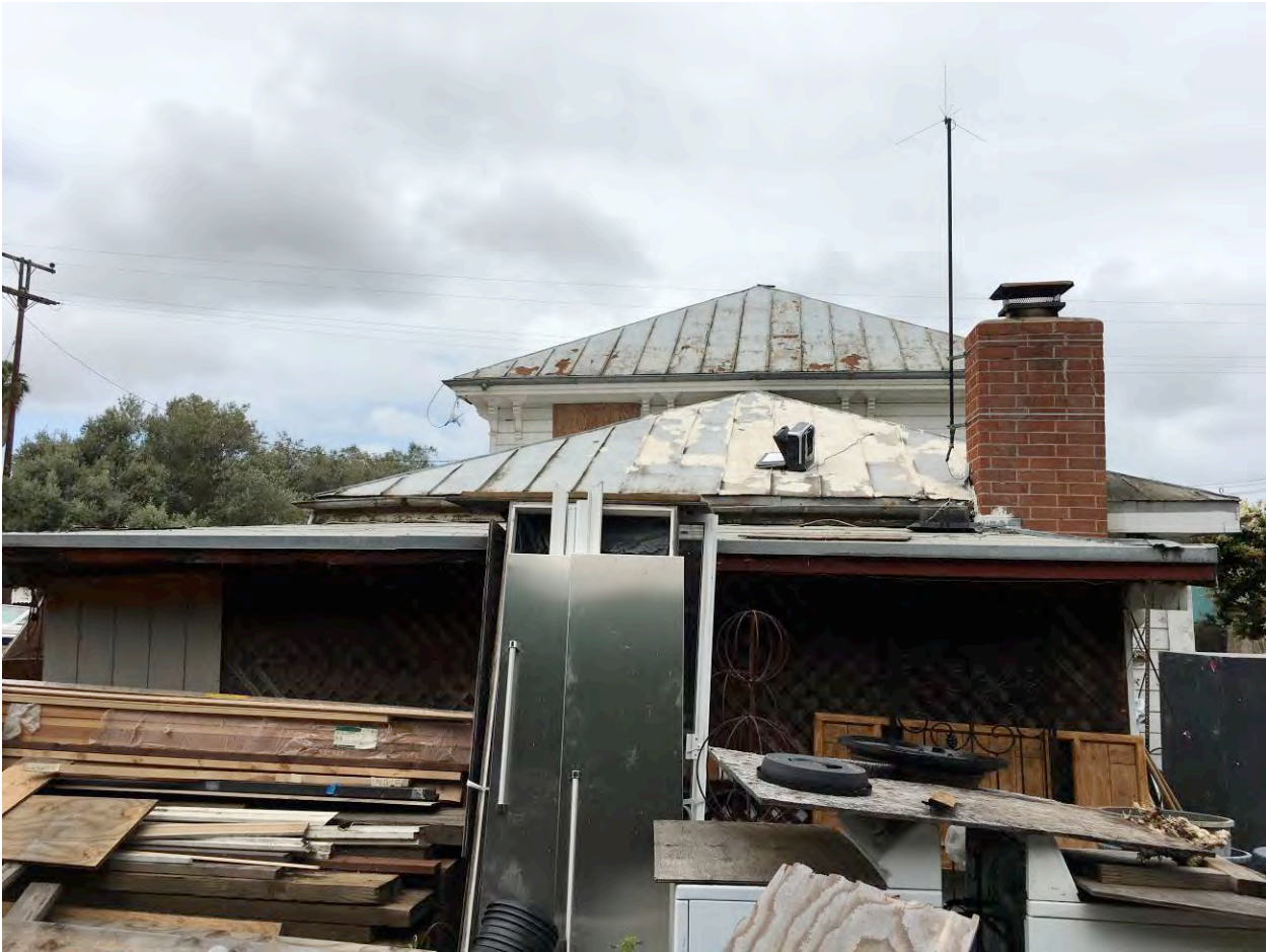
Photo 5: View west of the east wing, east facade.
