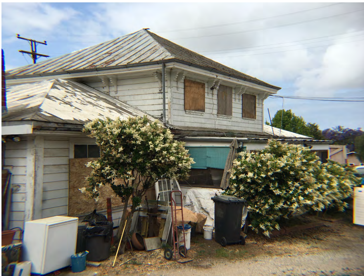
Photo 1: View southwest of the front elevation.
