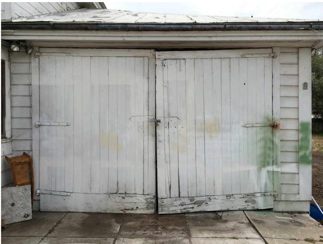
Photo 18: West wing garage doors.
