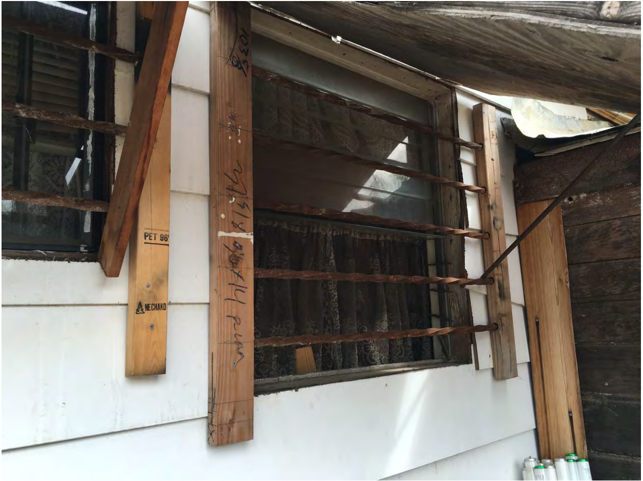
Photo 13: Opening / window detail at the south elevation.
