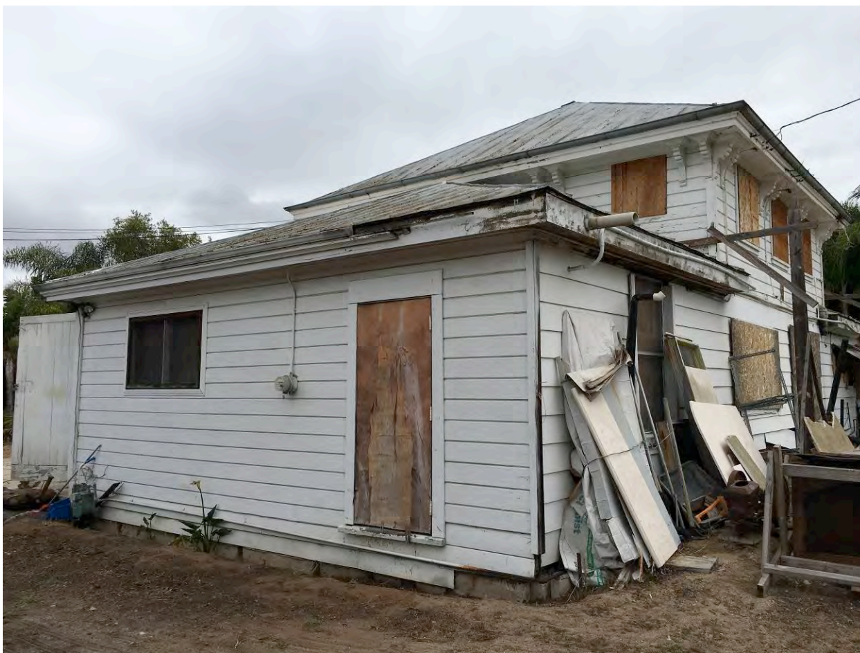
Photo 15: View of the southwest corner at the west wing.
