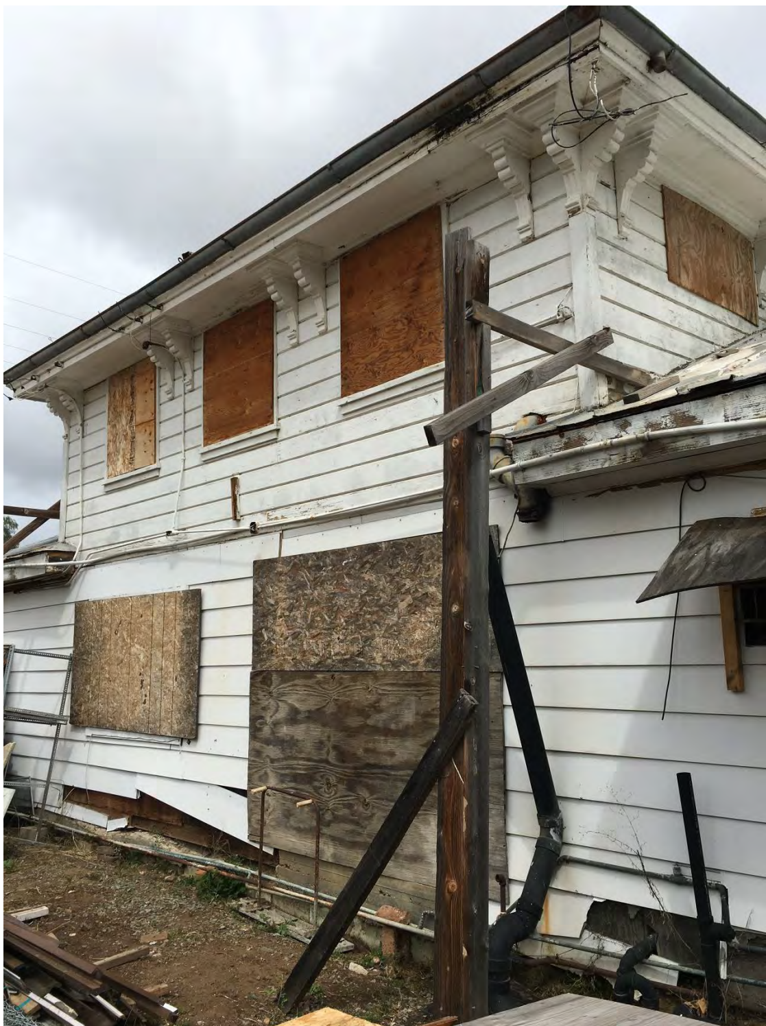
Photo 14: South elevation central block.
