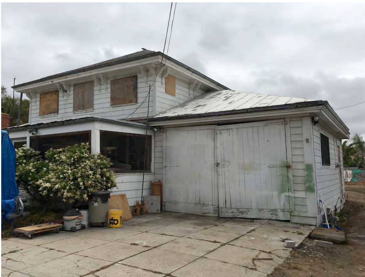
Photo 16: View south of the north elevation with the west wing in the foreground.
