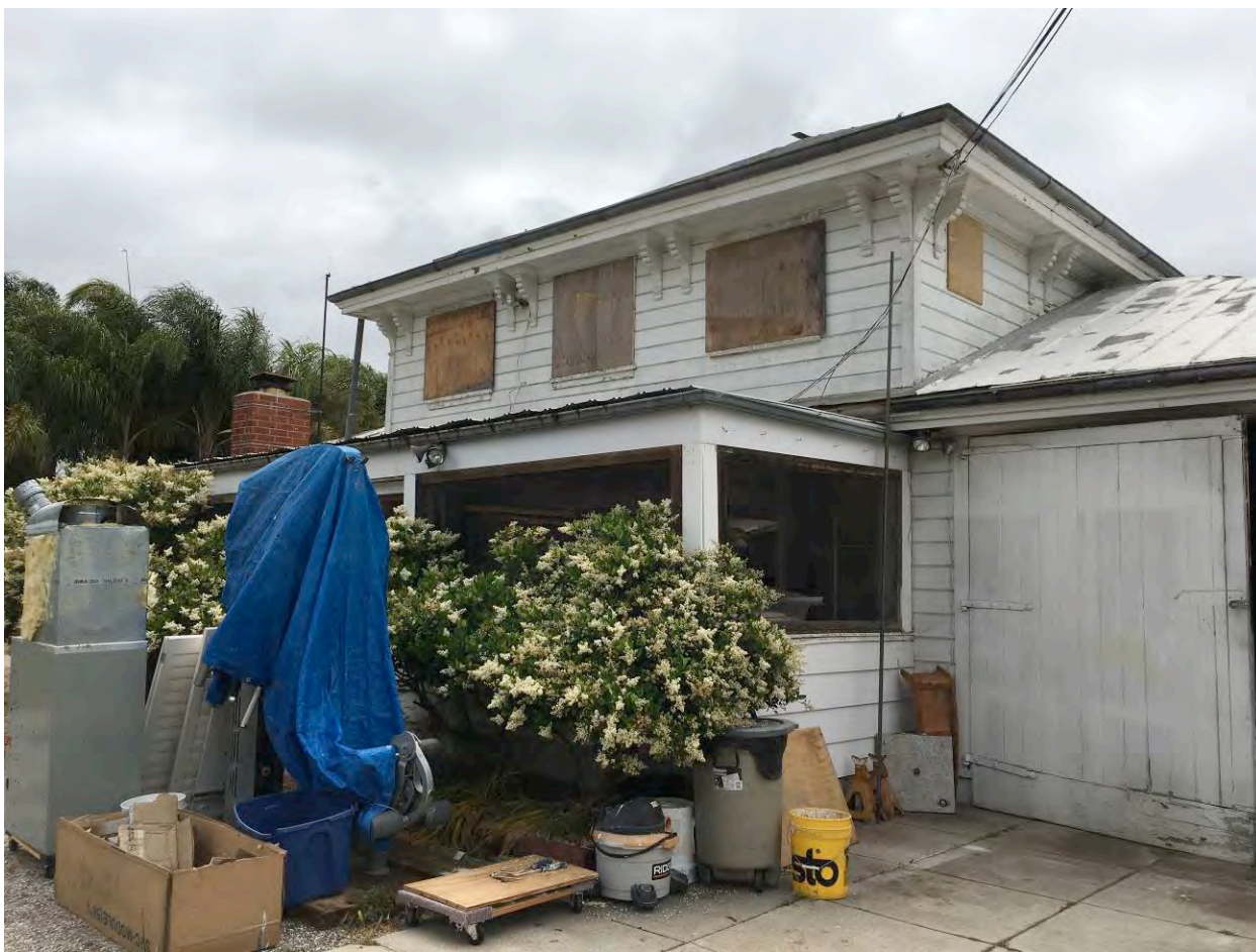
Photo 21: View southeast of the north elevation.
