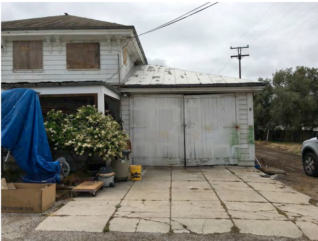
Photo 17: View south of the west wing.
