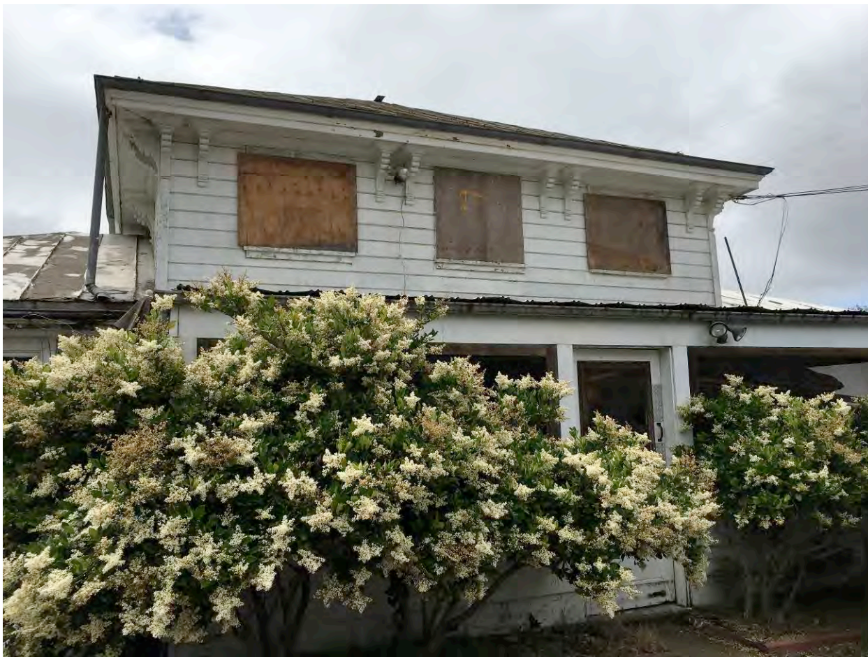
Photo 22: View south of the north elevation, central block.
