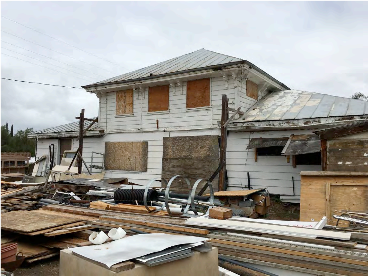
Photo 9: View north of the south elevation.
