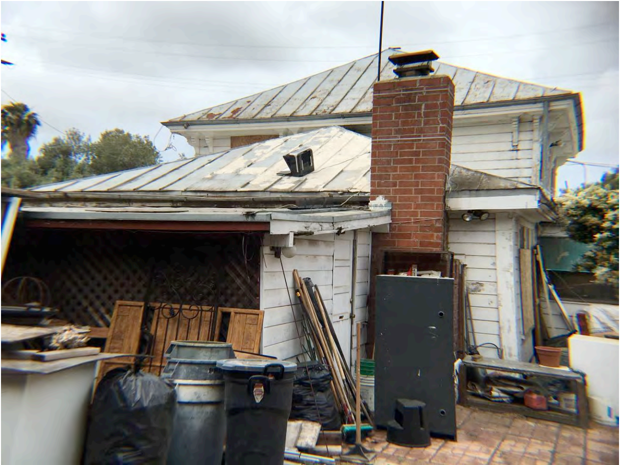
Photo 4: View west of the east wing, east facade.
