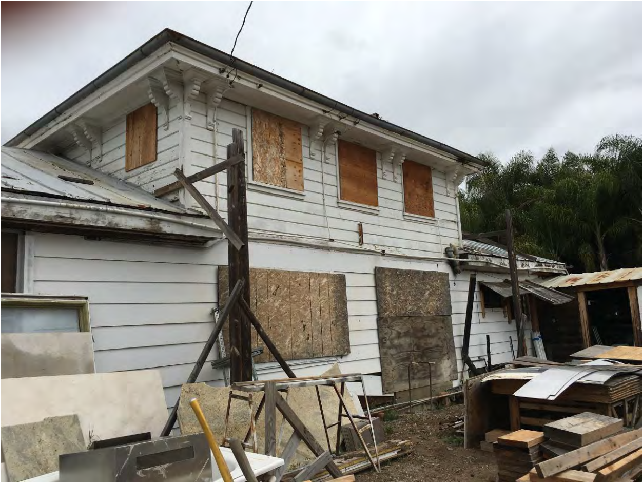
Photo 11: View northeast of the south elevation.
