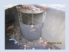
Drainage Insert (grate inlet style)
